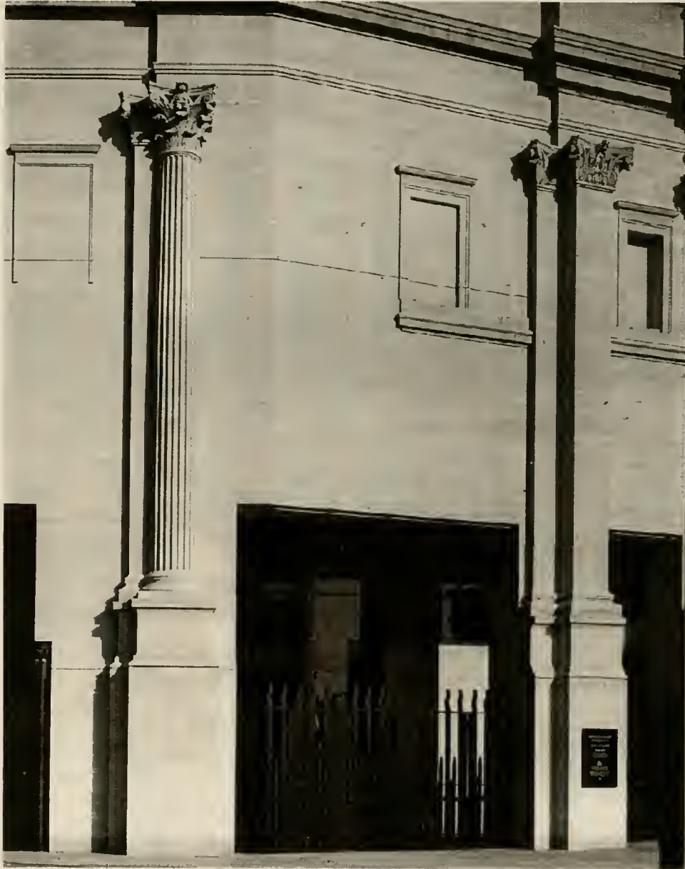
Fig. 4.13 – Single column on Sainsbury Wing façade.
